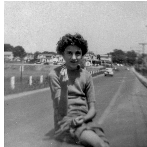
Sally Moore W Sixth Ave Bridge
