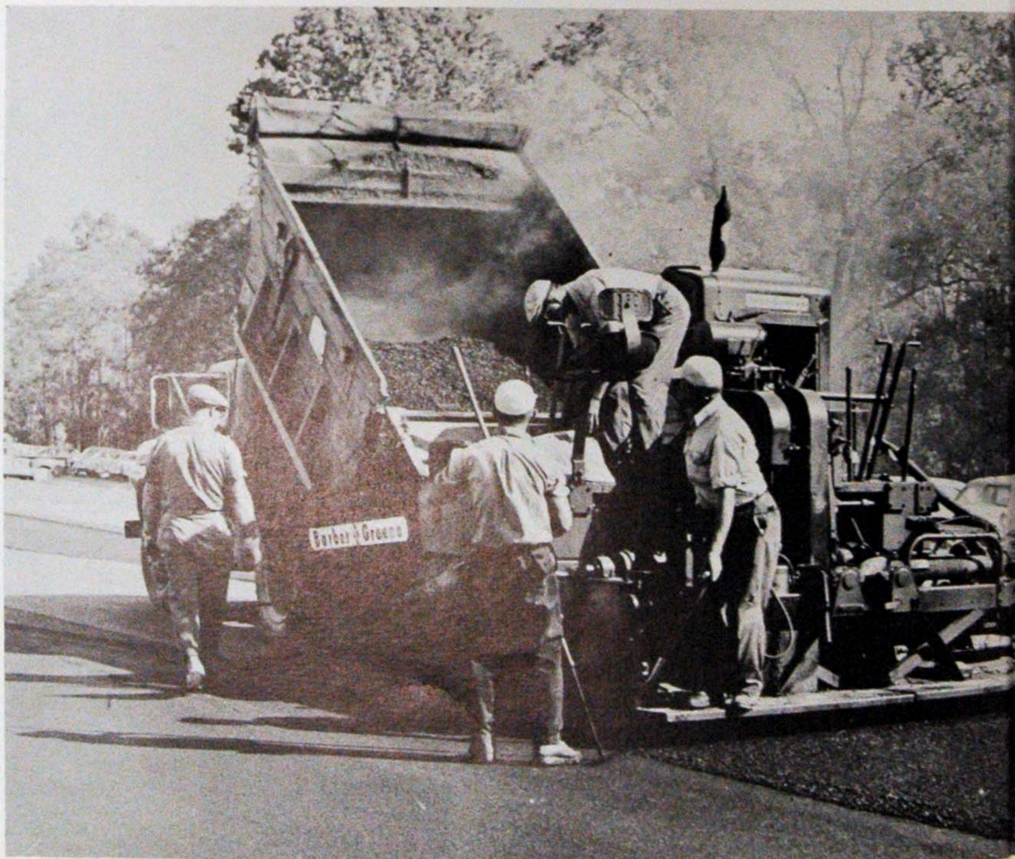
Workmen, as busy as a hive of bees, finished laying the asphalt in front of the school.
